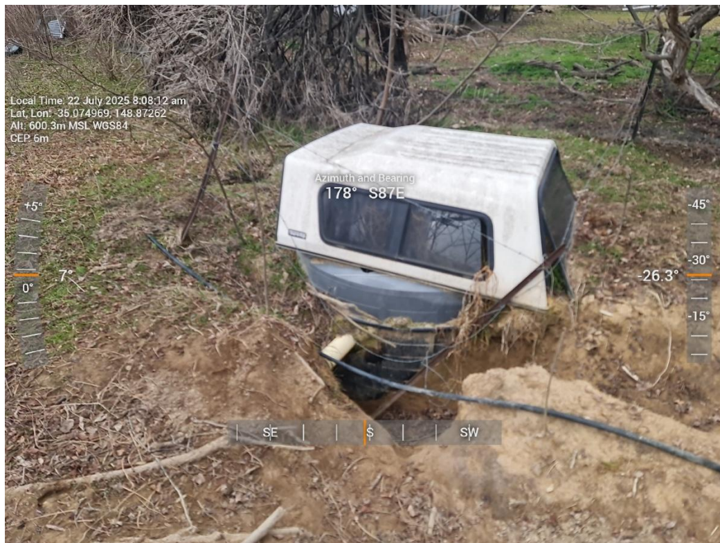
Figure 13: Existing septic tank servicing dwelling on proposed Lot A showing wombat damage.
